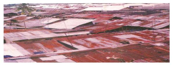
Plate 2. Cluster of zinc roofs with various degree of rusting/caving-in
